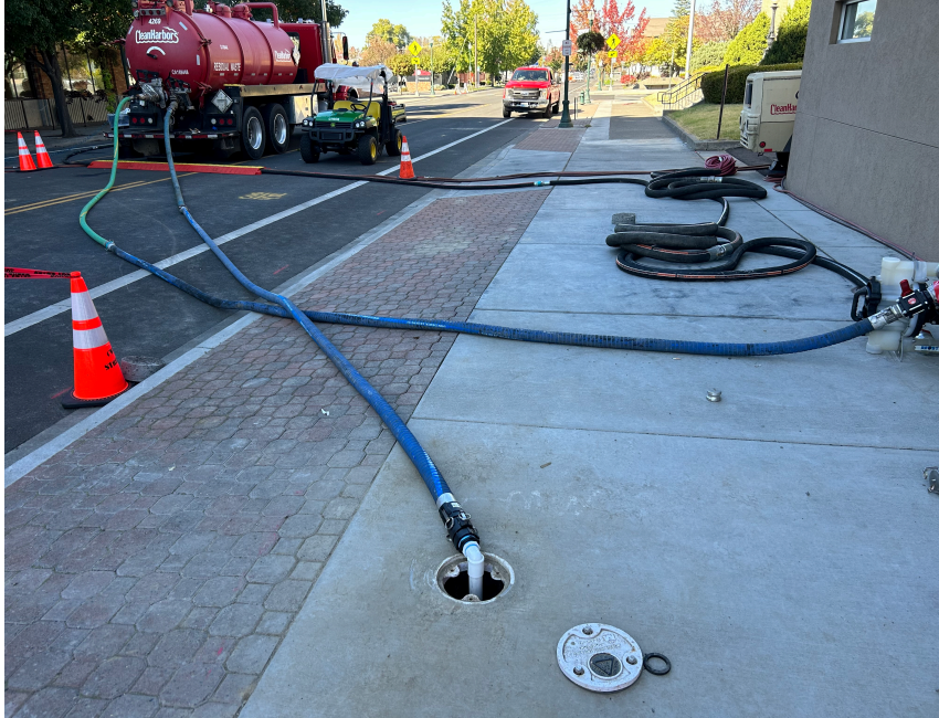
Groundwater monitoring well contamination extraction operation.
